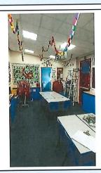
Plasterboard ceiling above suspended ceiling, plaster skim to brick walls and concrete floor beneath
