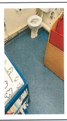
Plaster skim to plasterboard and brick walls partly ceramic tiled. Ceramic toilet cistern and plastic seat.
