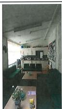
Plaster skim to plasterboard and brick walls and concrete floor beneath modern vinyl and carpet. Glass
