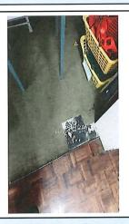
Low damage: a few scratches or surface marks, broken edges on boards, tiles etc. Green floor tiles and bitumen adhesive to concrete floor.
