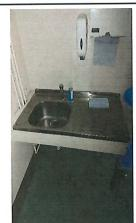
Low damage: a few scratches or surface marks, broken edges on boards, tiles etc. Recommendations Bitumen sink pad to the underside of the sink unit.
