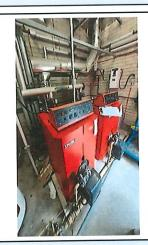
Modern boilers x 2 and mmmf insulation to pipework beneath metal cladding. Modern metal flue pipe.
