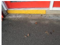
Good use of nosing to highlight step up
